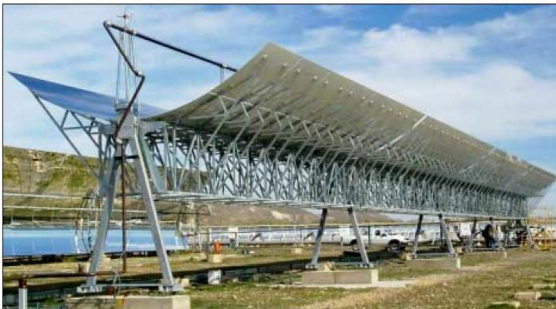
*Figura 52: Prototipo de captador EUROTROUGH, en la Plataforma Solar de Almería (fuente: Development of a Low Cost European Parabolic Trough Collector - EUROTrough, Research funded in part by the European Comission, in the framework of the Non Nuclear Energy Programme JOULE III)*
