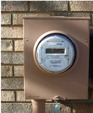
Source: MySmartGridHome (Reid, 2009) This image shows the Boulder smart meter.
