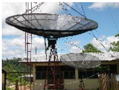
Figure 18. Radio antenna installed. Source: EsF
