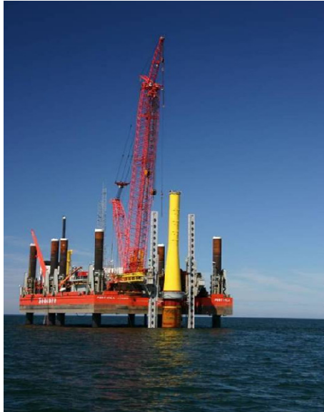
Figure 2.36 Pile lift and reorientation
