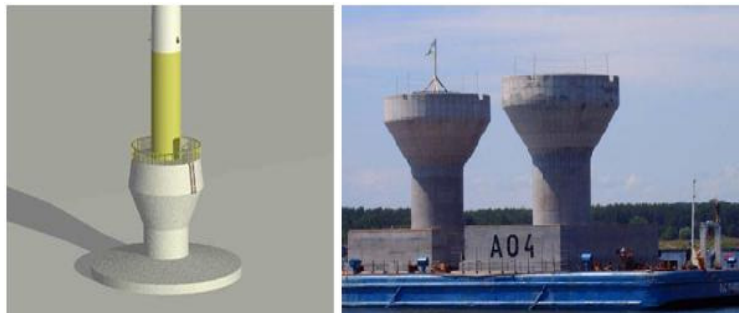
Figure 6. Gravity foundations
