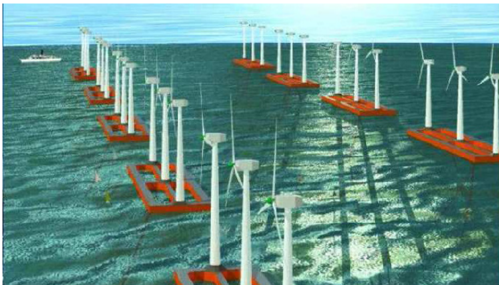
Figure 2.20 Stabilized floating support structures
