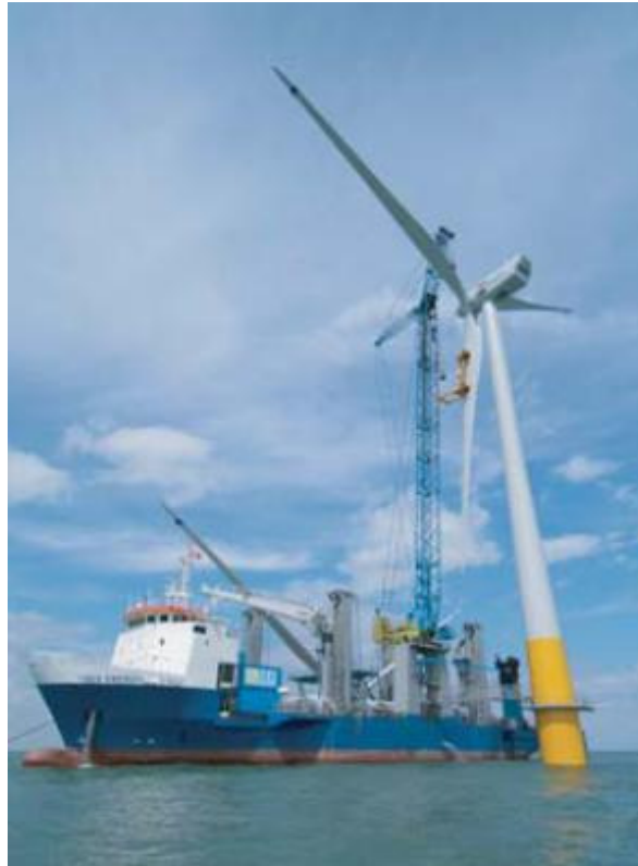
Figure 2.40 Turbine installation
