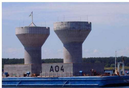
Figure 2.8 Concrete gravity foundations at Lillgrund, Sweden
