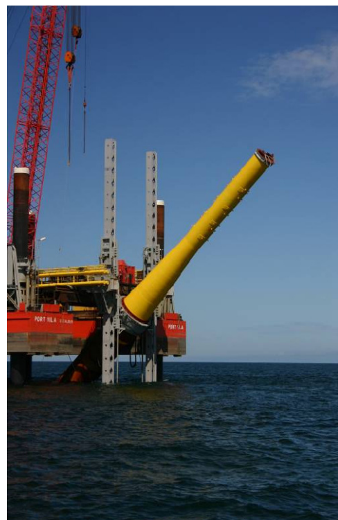
Figure 2.35 Initial pile lift
