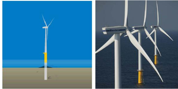
Figure 7. Monopile foundations
