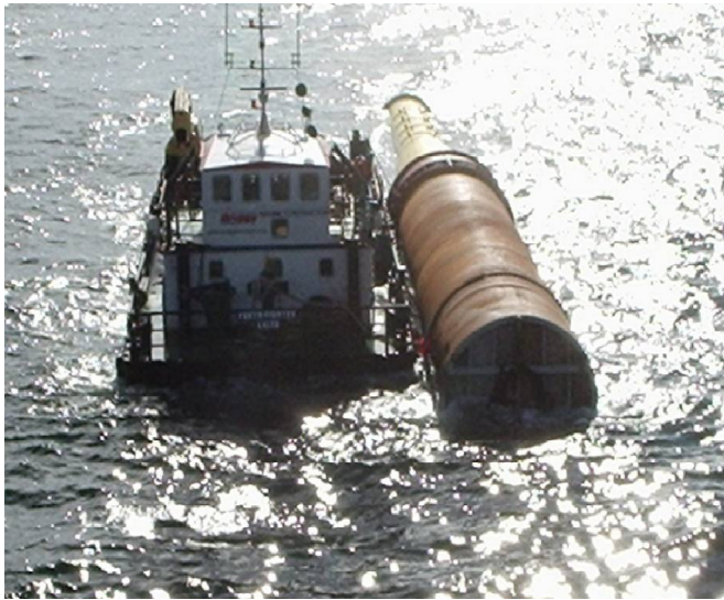
Figure. 2.33 Pile towing
