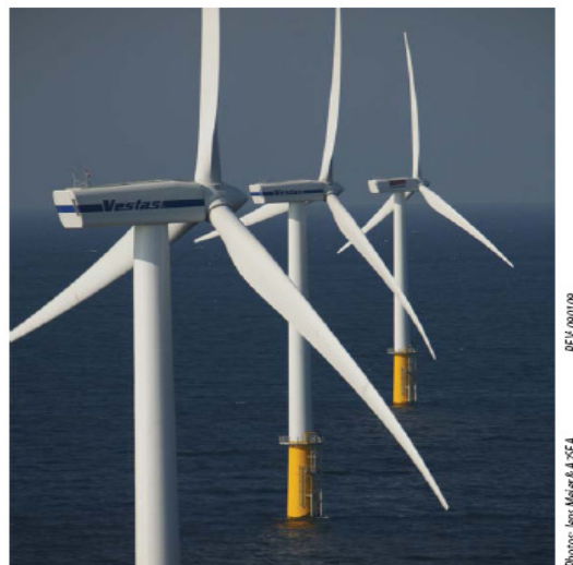
Figure 2.12 Q7 Wind farm with monopile foundations
